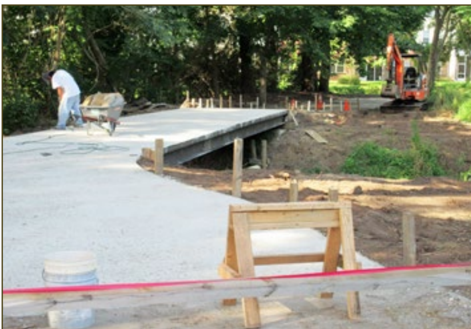
NEW BRIDGE BETWEEN NORMAN #2 GREEN AND #3 TEE
