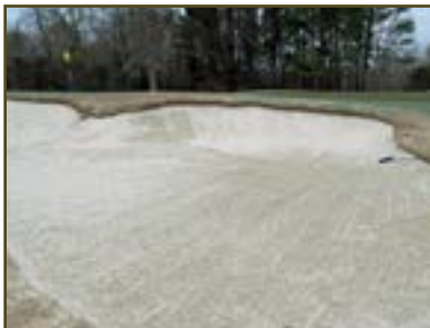
MAINTENANCE RENOVATED THE GREENSIDE BUNKER ON LOVE HOLE NO. 1
